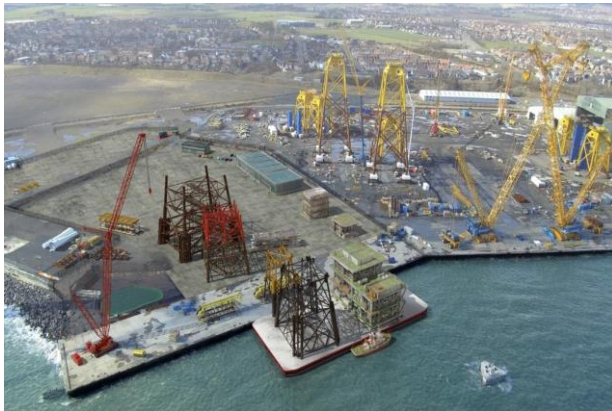
CessCom Decom EPF Decom Facility, Methil
