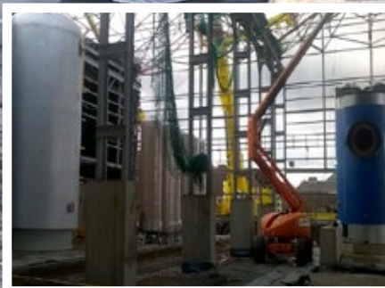
Thermal stores & heat exchanger
